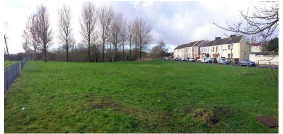
Fig 1 Cambrian North Basin before construction (February 2016)
