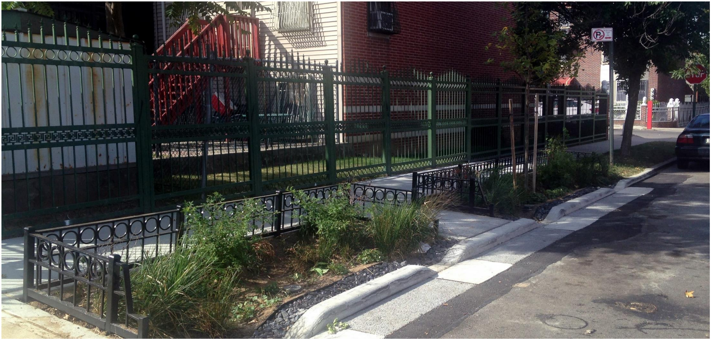
Bioswales constructed from the Newtown Creek contract
