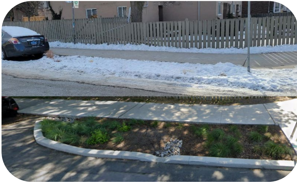
Carr Ave & Ryerson Ave Bioretention Bumpout NO Visibility during winter.
