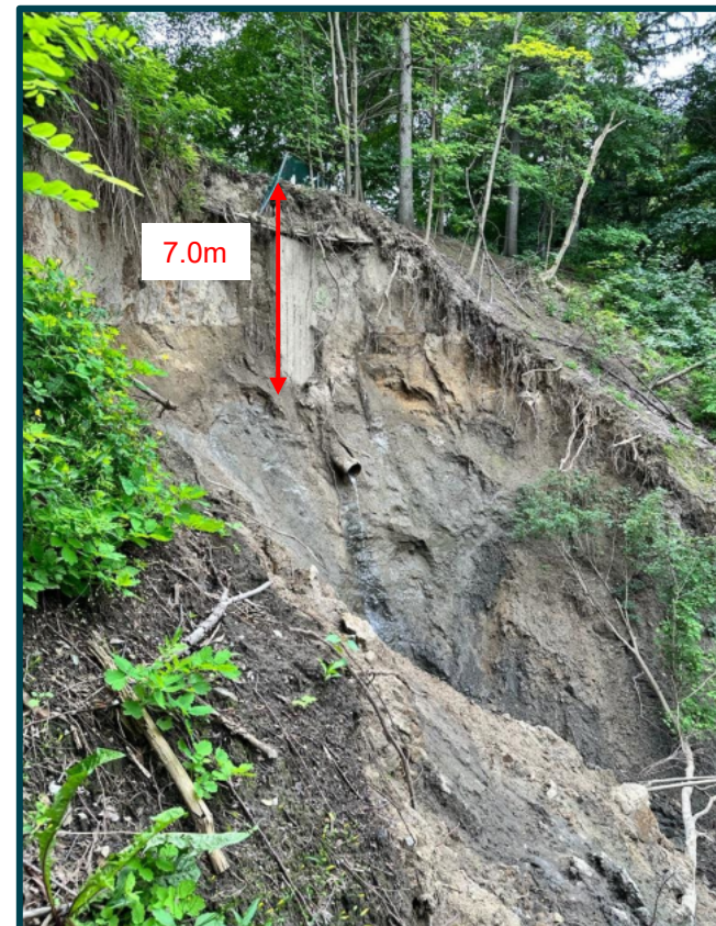
Maintenance Hole at Risk of Failure
