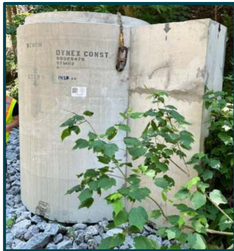
Precast MH c/w External Drop
